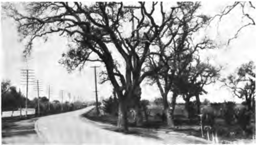
State Highway in Santa Clara County.
